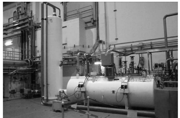
Fig. 8. Cryogenic moderator system refrigeration system showing the new vacuum enclosure used for a vertical orientation of the heat exchanger.
